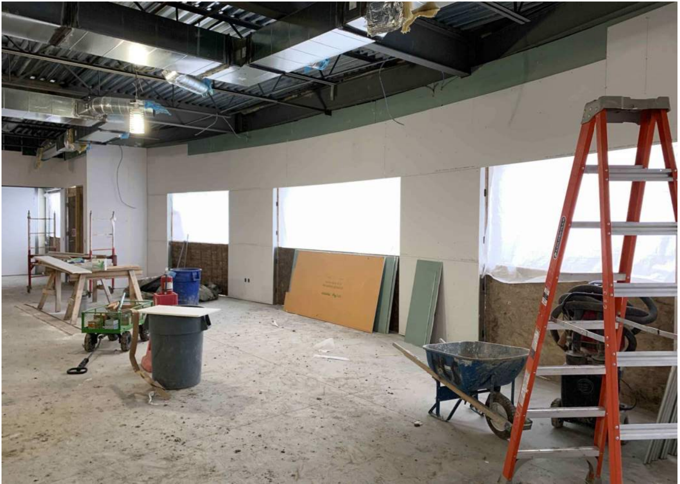
Interior drywall at the media center.
