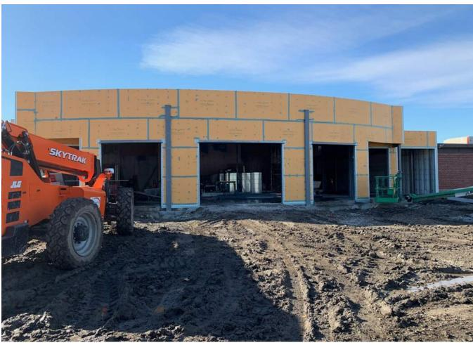
Laying block walls that were removed in order to set new steel.
