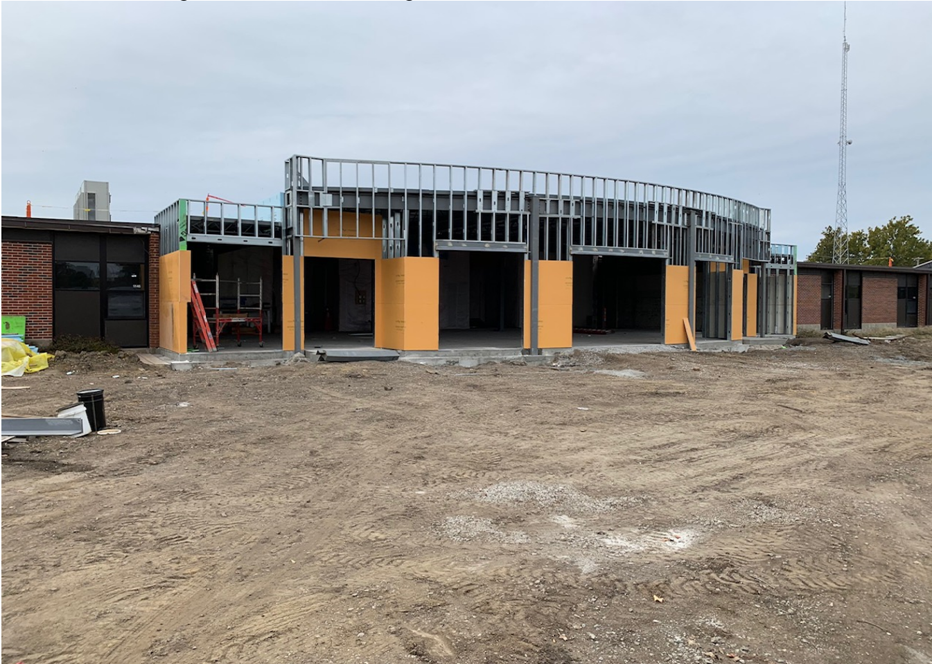
Metal stud framing and exterior sheathing.
