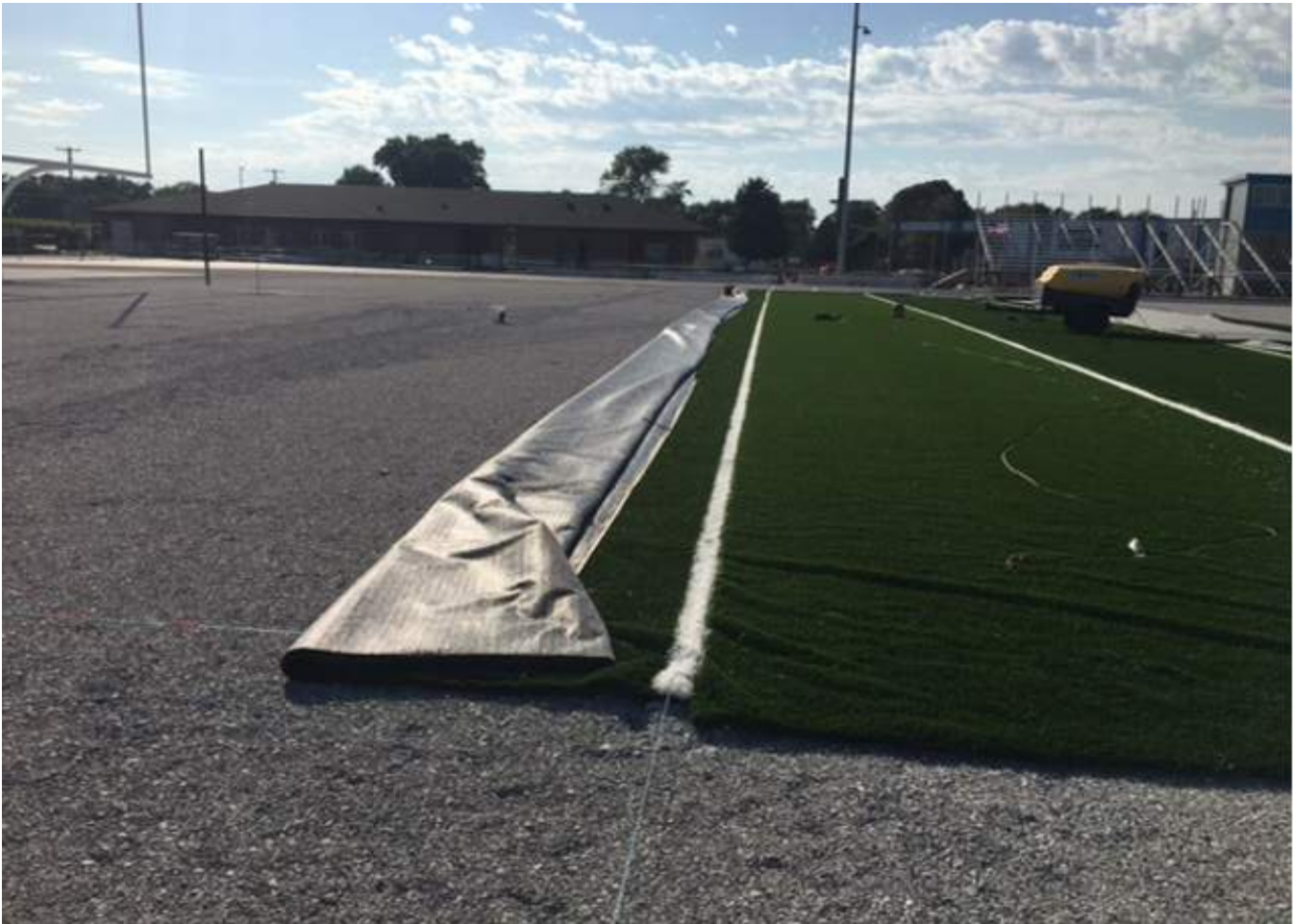
Start of turf installation.
